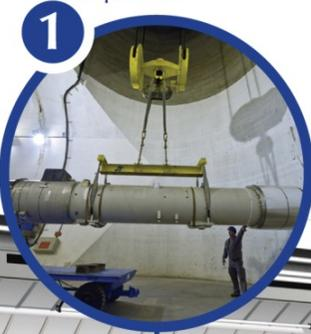
39 dipole magnets replaced
